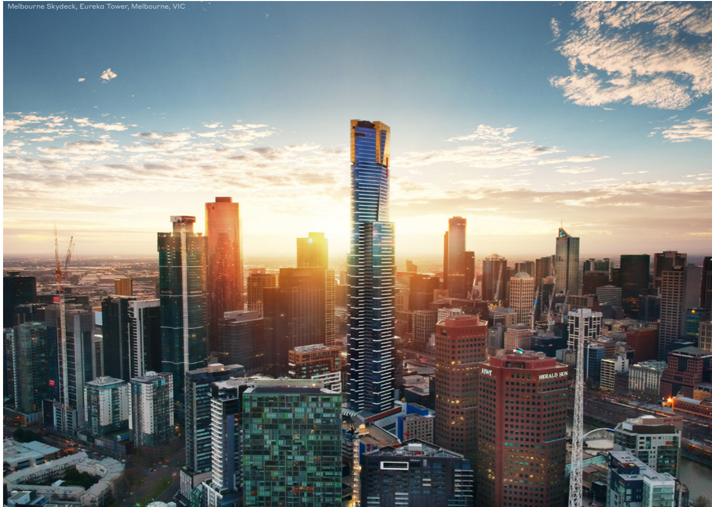
Melbourne Skydeck, Eureka Tower, Melbourne, VIC
